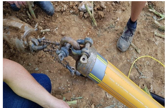
Attach small anchor shackle to duct pulling eye and secure with anchor pin.
